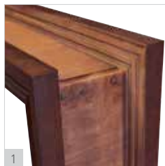
1 Jamb predrilled and secured with screws
